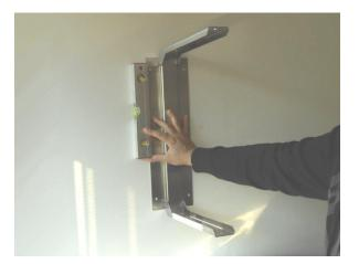
2) Drill the holes using screws and dowels that can support the weight of the MAXIReel according to the type of bracket used.
